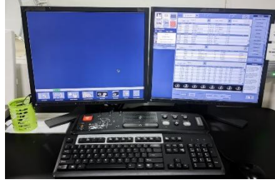
Gambar 5. Computer dan Operator Console (Instalasi RadiologiX RS Indriati Solo Baru, 2026)
